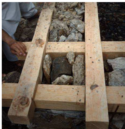
Figure 4. Configuration of bhatar bands and stone masonry.
